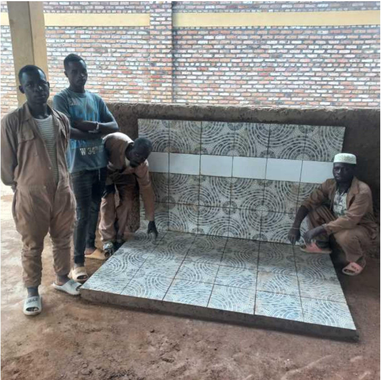
Figure 19 during practice of building tile
