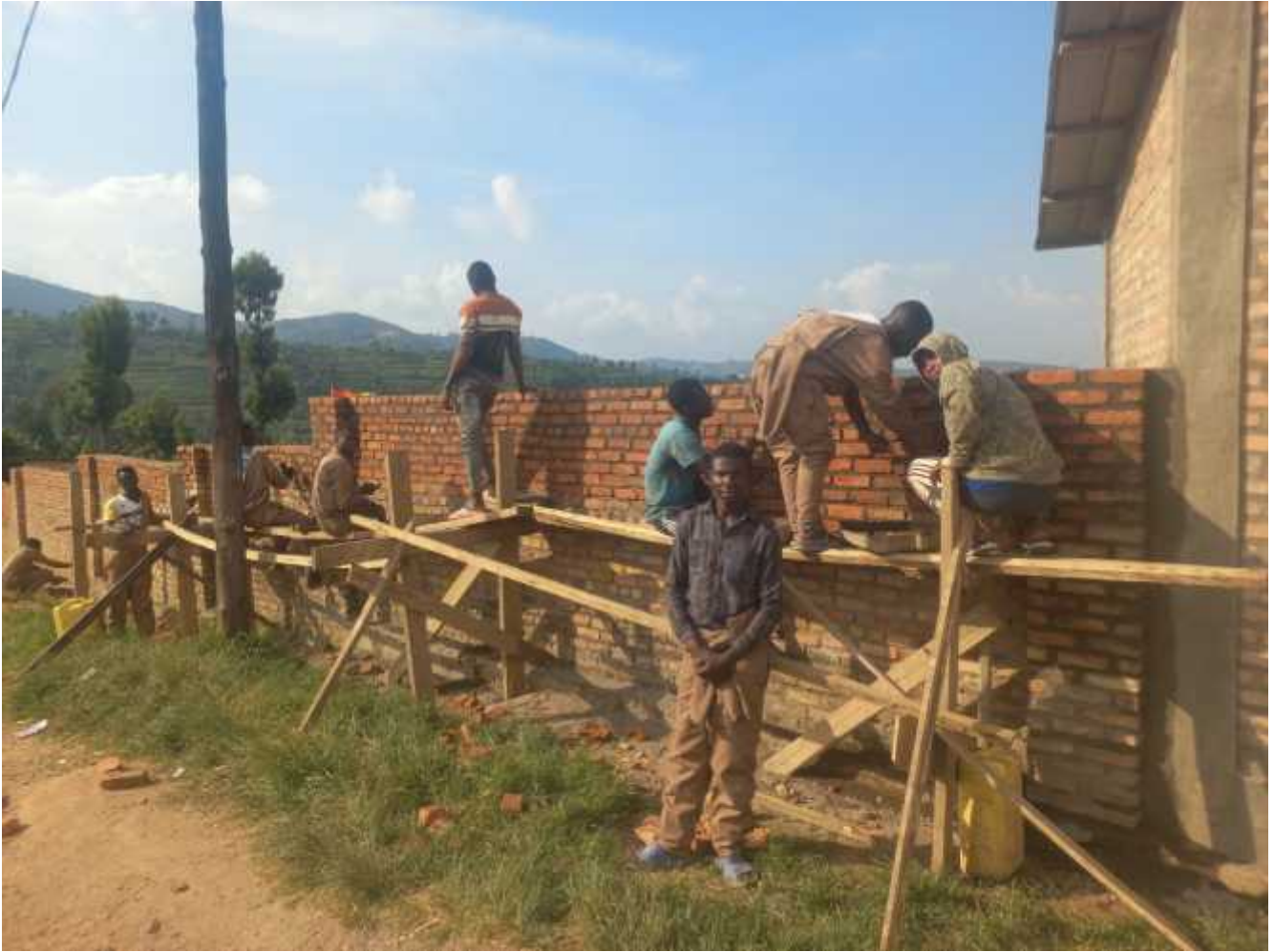
Figure 21 Students learning construction
